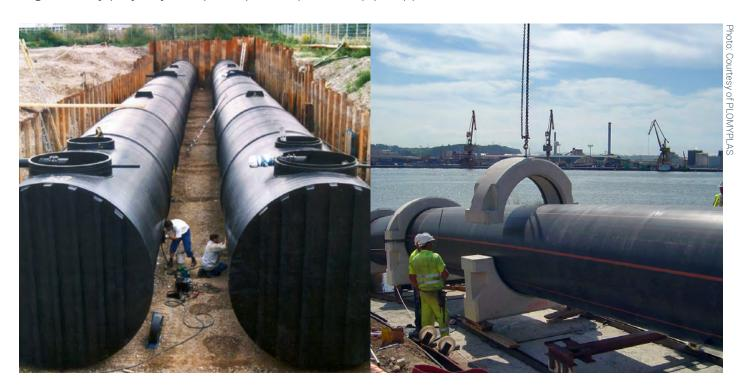
Hostalen CRP 100 black is a high density polyethylene (HDPE) PE 100 compound for pipes and fittings, which has steadily replaced traditional materials such as cast iron, ductile iron and concrete in piping systems. Smaller pipes can be coiled and installed over long distances without connections.
